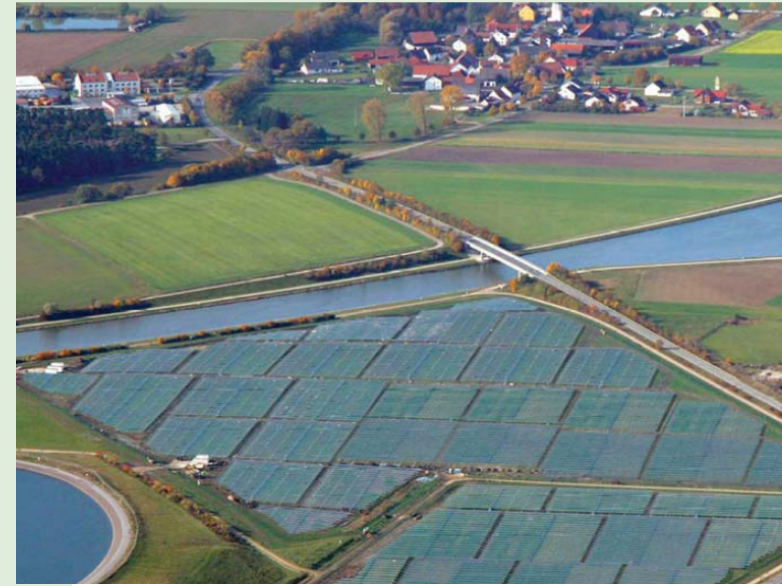
Central-Station PV: 6.3-MW Solarpark Mühlhausen (Credit: SunPower)
