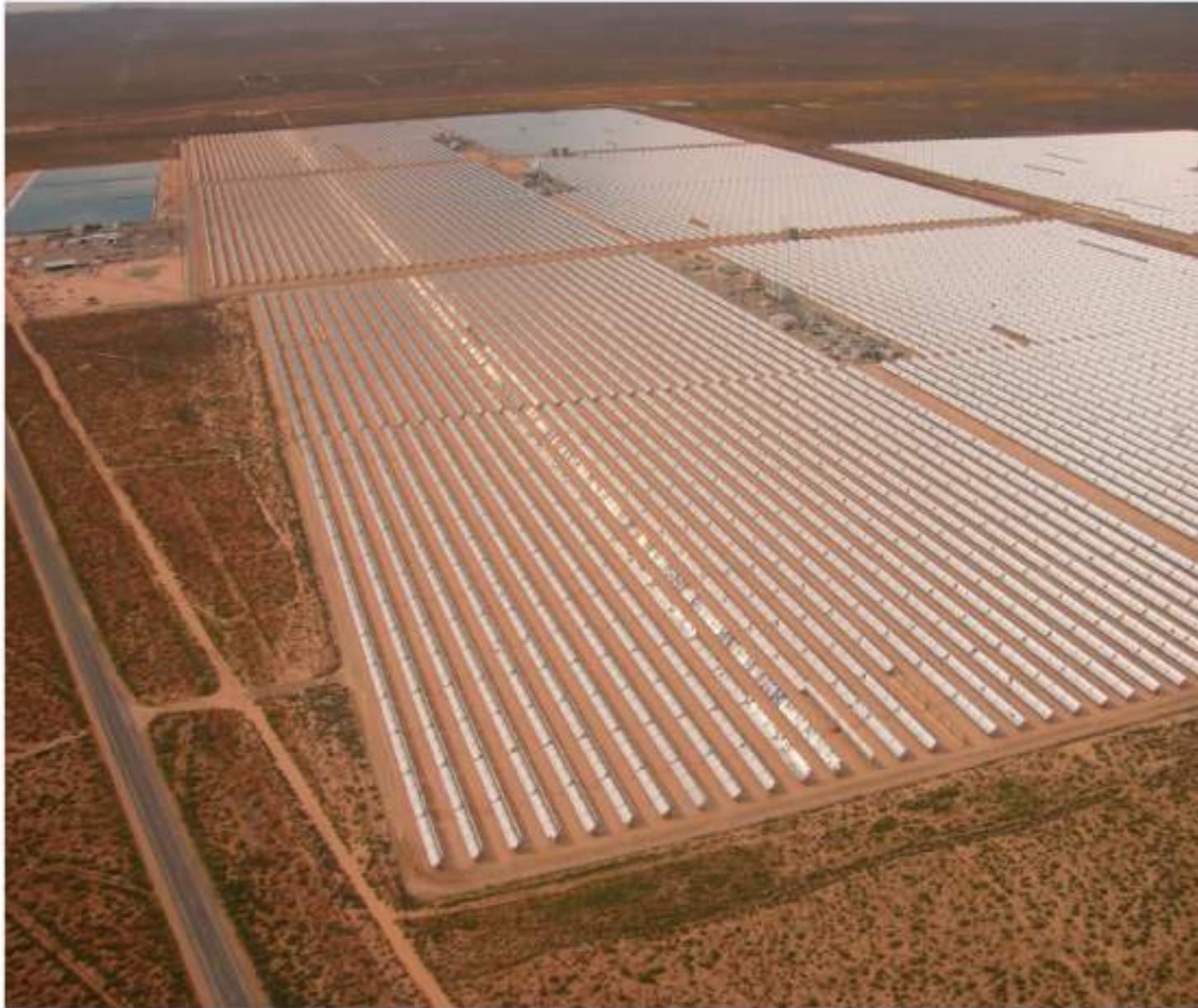
Figure 9. Parabolic trough CSP plants (such as the one in California, pictured here) utilize a mature technology; 419 MW of capacity are currently operating in the U.S., while several 50-MW plants are under construction in Spain. Source: Alan Radecki.
