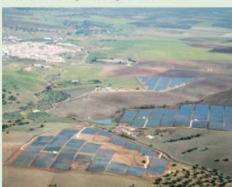
Central Station Tracking PV in Portugal (Credit: SunPower)
