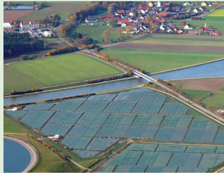
Central-Station PV: 6.3-MW Solarpark Mühlhausen (Credit: SunPower)
